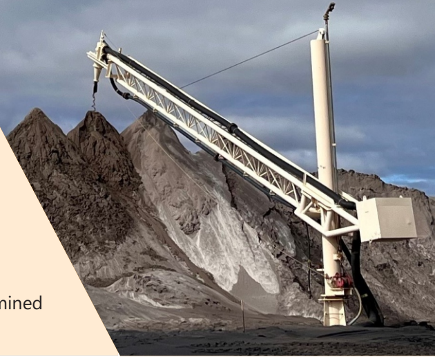
HMC stockpile ready to be transported to Picton
