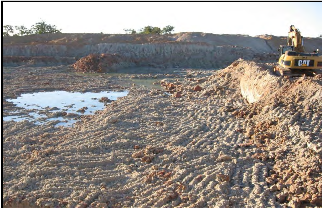
Plate 2: Water will re-infiltrate the Aquifer through Drainage Channels Constructed around the Perimeter of the Pits
