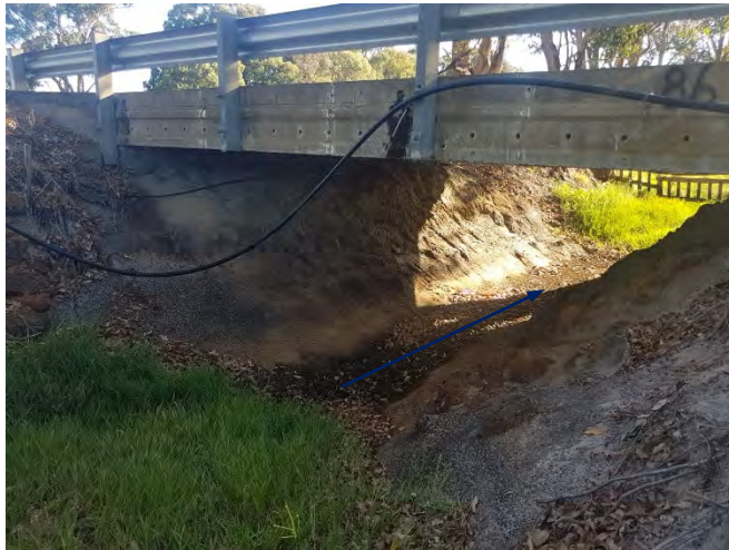
2. WC Bridge 86, looking West
