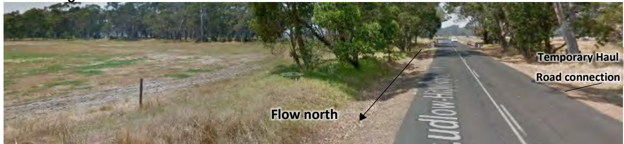
3. Looking south along Ludlow-Hithergreen Rd at WC Bridge 86
