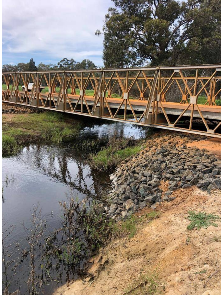
Figure 2: Abba River post bridge installation with rock pitching
