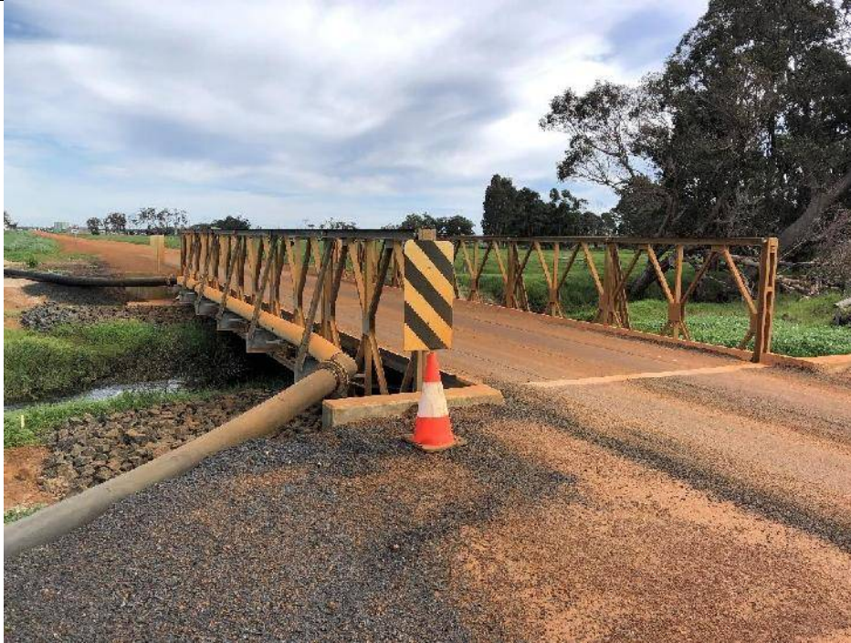
Figure 3: 23m of bitument installed either side of bridge
